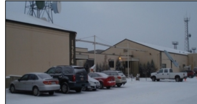
Current Mission Control Center is located in two 74 year old converted warehouses with mechanical systems that are inadequate to maintain required temperatures.
